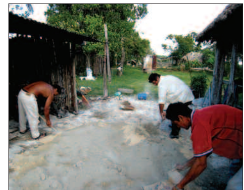
Rebuilding in Belize after Hurricane Dean
